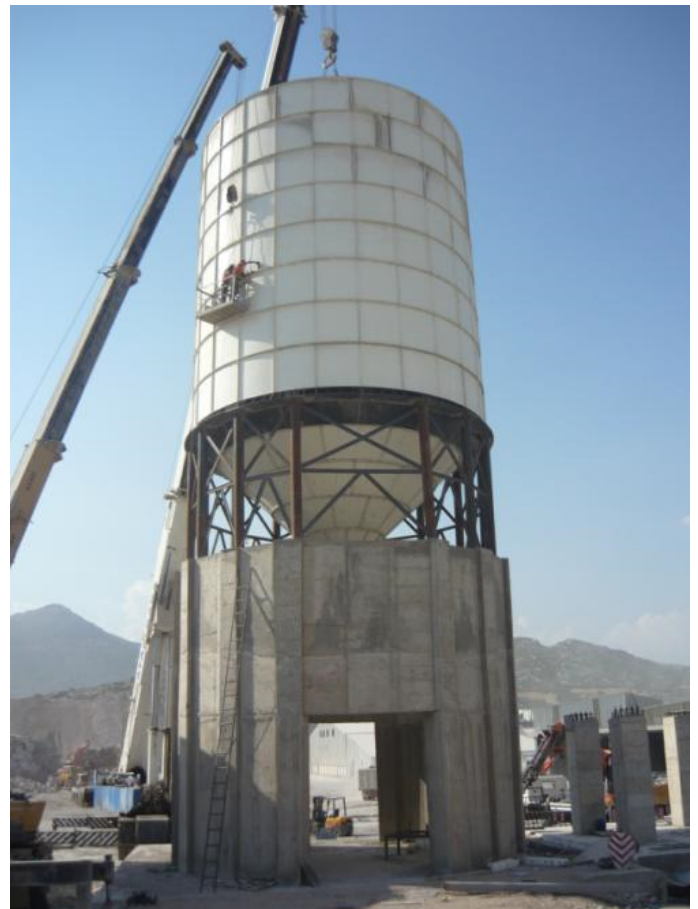
Figure 5: 1,000 ton capacity silo. This particular silo, manufactured by Zimmerman Industries, is 70 ft. tall, 27 ft. in diameter, and weighs 8 tons.
